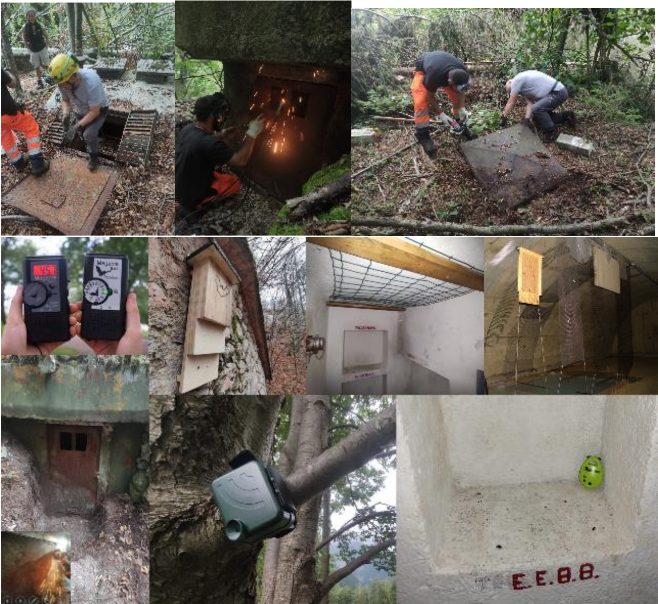
Fig. 9 Restoration activities on bunkers, monitoring equipment and bat-friendly structures installation.
